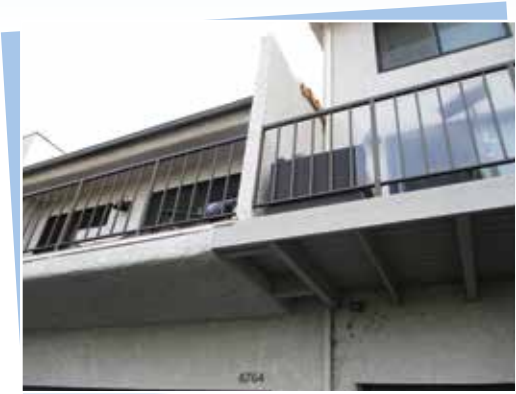
Wood framed, elevated, railings subject to fallibility; inspection requirements likely apply
