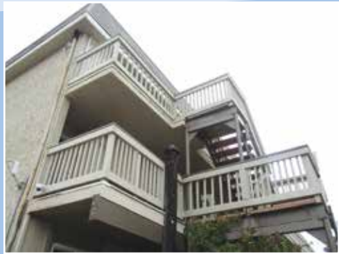
Metal framed stairs likely exempted; however, decks are wood framed, elevated inspection requirements likely apply
