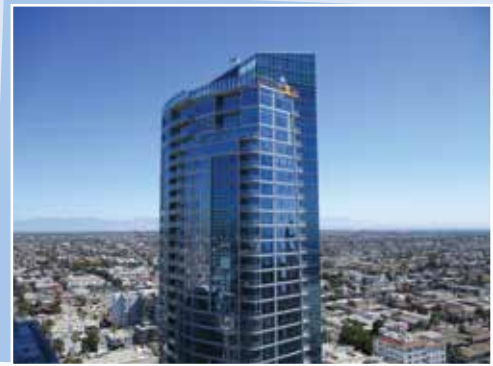
Concrete and steel construction; elevated inspection requirements likely does not apply. Railing should still be inspected regularly.
