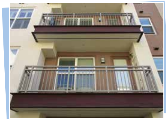
Wood framed, elevated, railings subject to fallibility. Note the presence of ventilation; inspection requirements likely apply
