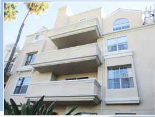
Wood framed, elevated, railings subject to fallibility; inspection requirements likely apply
