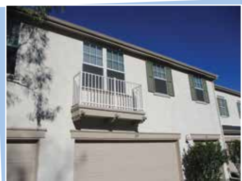
Decorative element, not designed for human occupancy; elevated inspection requirements likely does not apply
